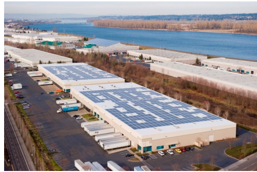
ProLogis / Portland Electric , Portland, Oregon, USA, 3.5 MWp
