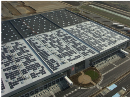
ProLogis, Moissy-Cramayel, France, 445 kWp
