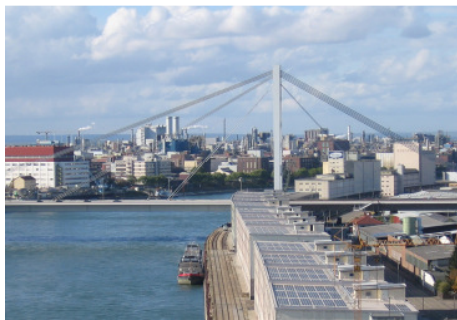
Port Authority Mannheim, Block I, II and III, Germany 370 kWp
