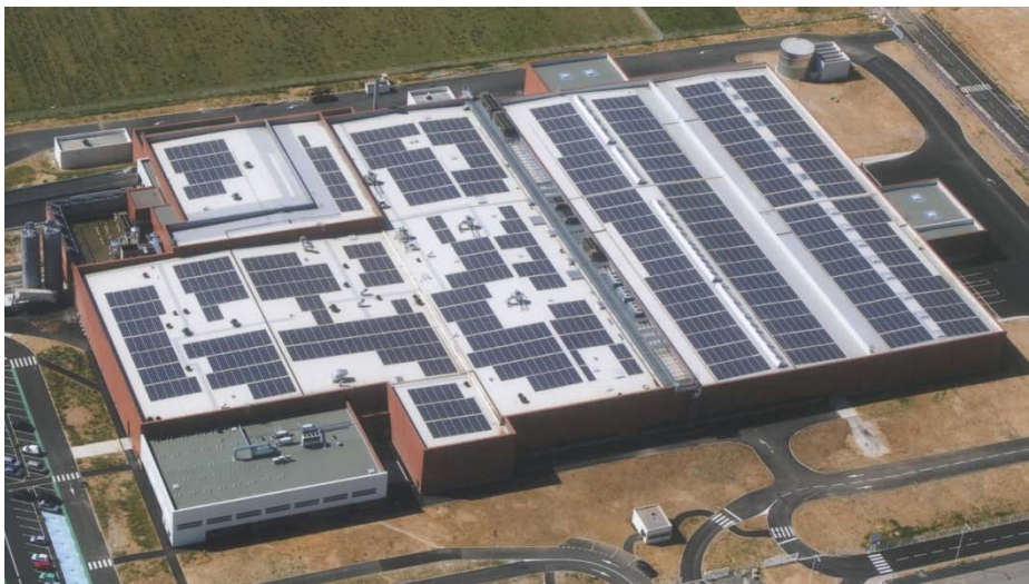
CEMOI Chocolatier, Perpignan, France, 550 kWp
